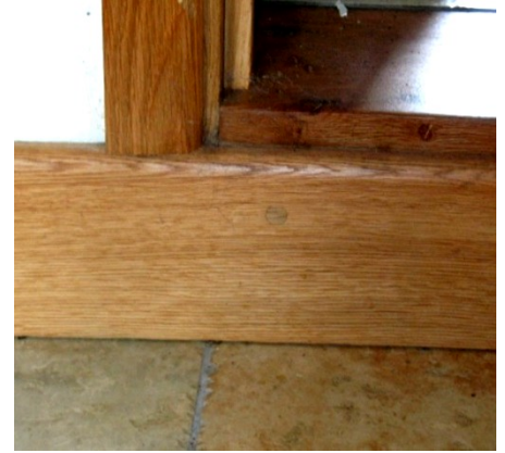
Nailed oak skirting
