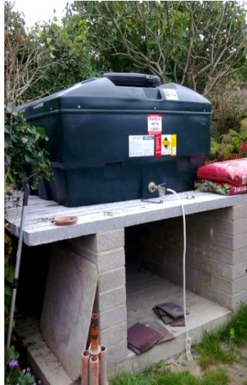
Oil tank above flood height
